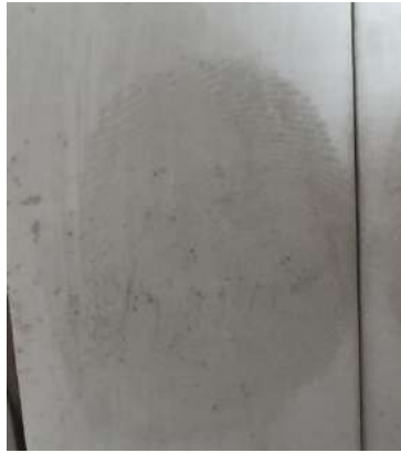
Figure 14: Mehandi powder on Switch board
